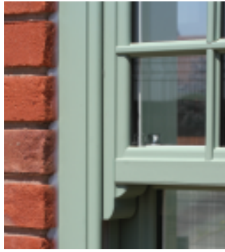
Run through sash horns
